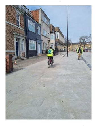
Pedestrians and cyclists will be directed on to the newly laid footpath on Howard Street to allow the construction team to begin installing the drainage channel on the eastern side of the street, including the creation of tree pits.
